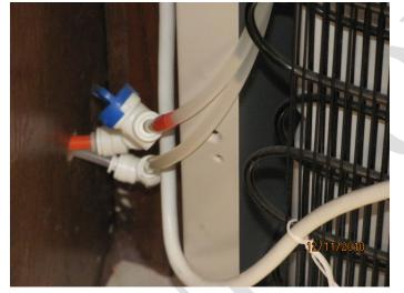
I have 2 lines coming through the cabinet because I'm running a line back to the refrigerator icemaker from my water filter (pictured below). My water cooler has a compartment under it so I put an inline water filter for the water cooler and the refrigerator icemaker.
