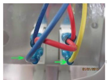
The green arrows are pointing to the wire of the switch that will be off when the switch is in the off position.
