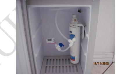
Water filter is not included in any of the kits offered. The type of water filter shown is a Culligan IC 1000.
