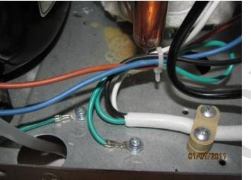
You can connect to the switch on the heater or the cooler side of the switch. The black wire coming from the power cord may change into another color wire going to the switch. My cooler black wire was spliced to a red wire that went to the hot and cold switches.
