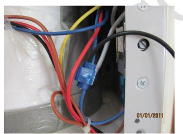
Connect the black wire quick connect to one side of the water solenoid valve wire.
